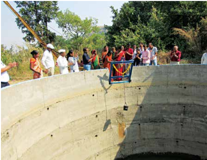
Well construction - Rural development project
